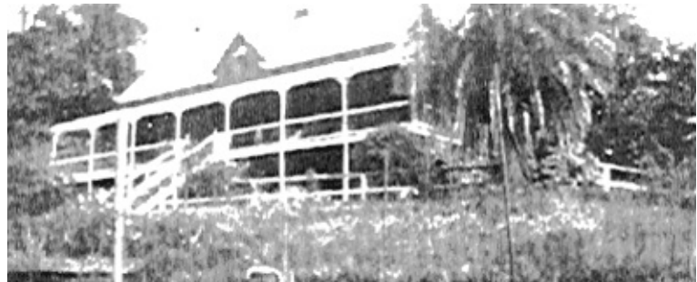
Picture 4. 24. James built this house at Corinda and called it Matavai .
