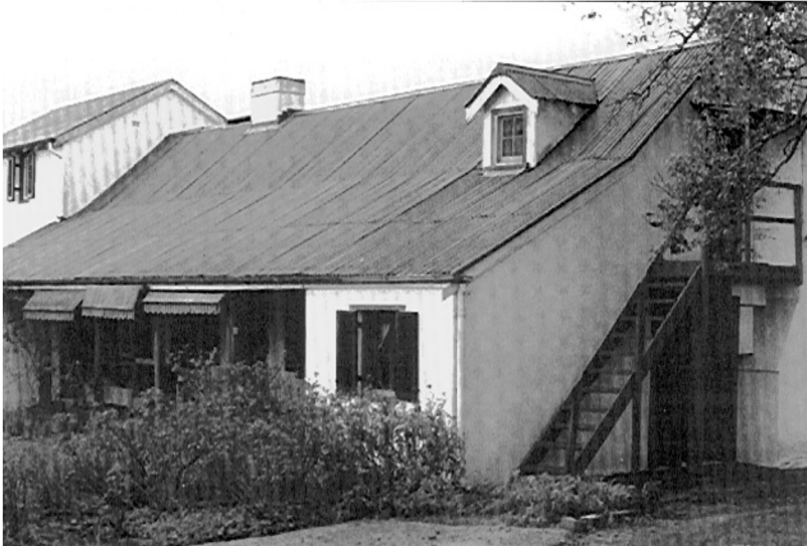
Picture 3. 12. This is Hassall Cottage, the original house built at Rowland's Macquarie Grove property of 400 acres granted to him by Governor Macquarie in 1810. Three years later Macquarie stayed there for two nights. The cottage was renovated in 1932 using materials from the original stables and has since been extended.
